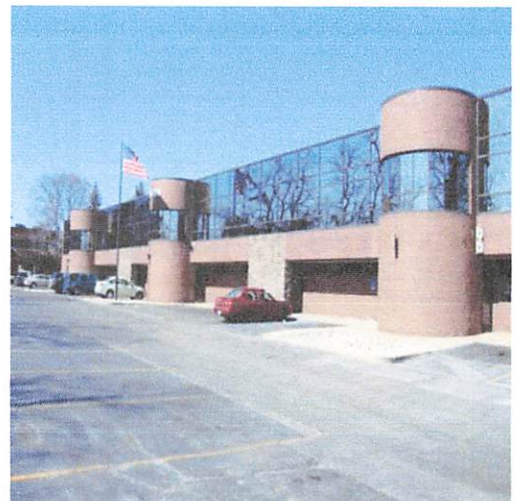
Front of building
